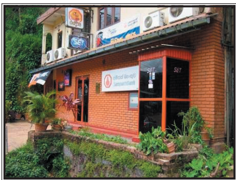
Typical Sampath Bank Branch to furnish community access and telecom hub. Photo by J. Metzger.
